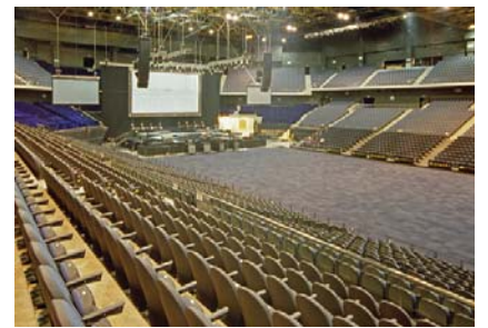
The new Venetian Hotel and on the burgeoning Cotai Strip entertainment district in the Chinese city of Macao features a high-performance sound system comprised of Meyer Sound MILO line array loudspeakers, 700-HP subwoofers, CQ-1 and UPA-1P loudspeakers, a Galileo loudspeaker management system and compact Meyer Sound M'elodie line array loudspeakers.
